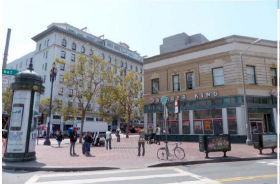
M40 – Civic Center Station Street Level Vent
