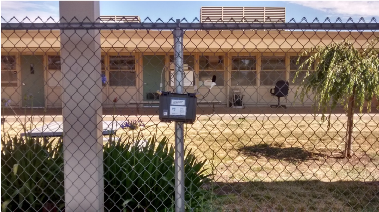
Figure B-5. Site LT-PH1: Oak Grove Middle School. 2050 Minert Road, Concord, CA (across street from “David/Minert” TPSS site)
