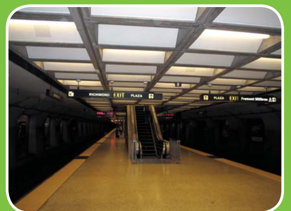
Dim Platform Lighting
