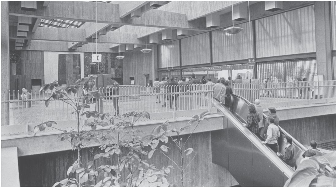
Pictured is Glen Park Station, which opened on November 5, 1973. The stations were located to connect central business districts throughout the Bay.
