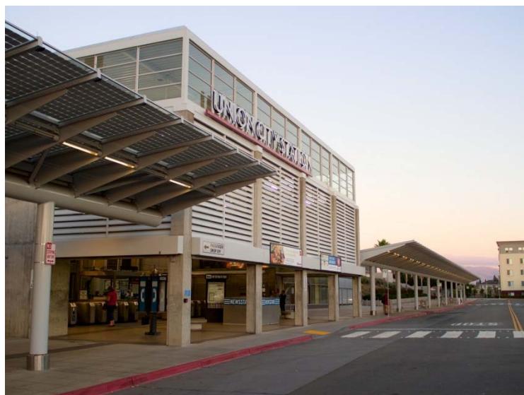
Figure 10 The recently completed improvements at the Union City BART Station highlights the goals of the Station Modernization Program. The project expanded access, improved the station environment, and facilitated multi-modal transfers, while upgrading the station appearance.
