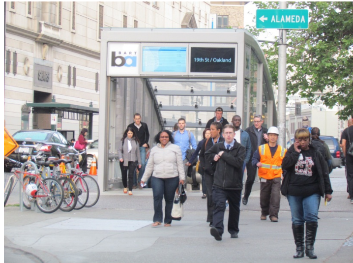
Figure 8 The recently completed enclosure over 20 th St entrance to the BART station in the morning rush hour, with the AC Transit Uptown Transit Center in the background. Currently no direct accessible connection exists between the BART Station and the Uptown Transit Center.
