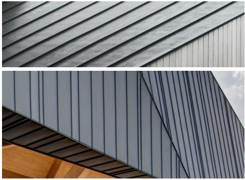
**Zinc alloy standing seam metal cladding:** standing seam metal is an extremely durable roof materials that can also be used for wall cladding. It is expressive of traditional craft yet can be used to clad contemporary, sculptural forms. The dark, neutral coloring of zinc alloy is both contemporary and neutral, and complements both the concrete of the existing station structure and the stucco and brick of the Transit Village.
