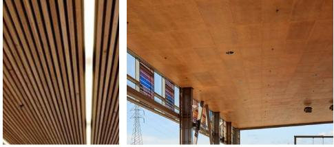
Wood-textured metal ceiling: while the use of natural wood remains controversial due to fire rating considerations, even a woodlike coloring or texture provides warmth and texture that is calming and uplifting.
