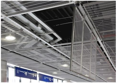
Metal mesh (metal fabric): while transparent to moisture and light, a metal mesh ceiling, if detailed correctly, can prevent pigeon roosting while providing a finished, clean surface. Where needed, access panes may be built into the ceiling system. Metal mesh or metal fabrics are also effective alternatives to glass fare barriers.
