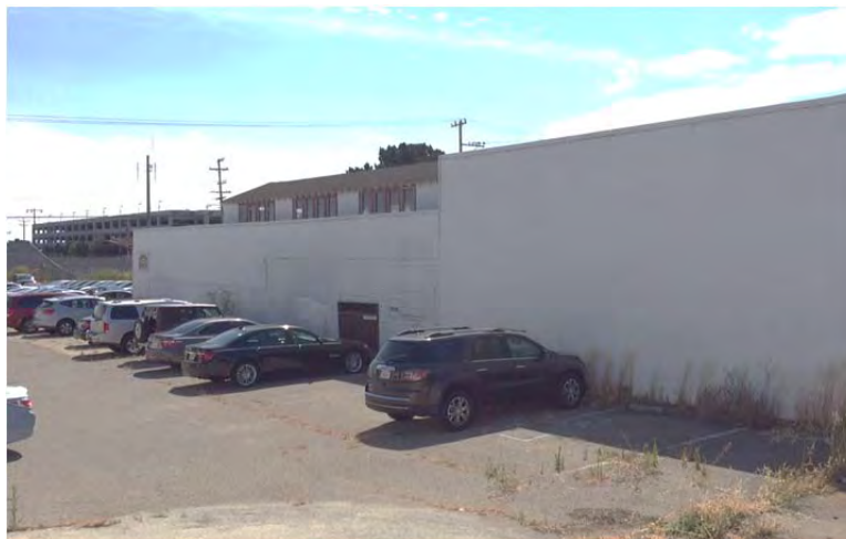
Side of building showing shop addition with clerestory windows.
