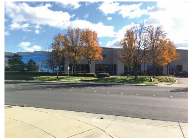
Commercial uses south of East Airway Boulevard.
