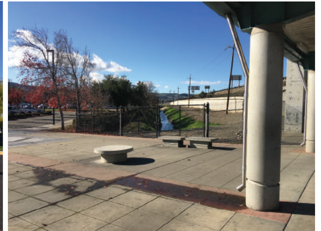
Chabot Canal immediately to the south of the Dublin/Pleasanton Station.
