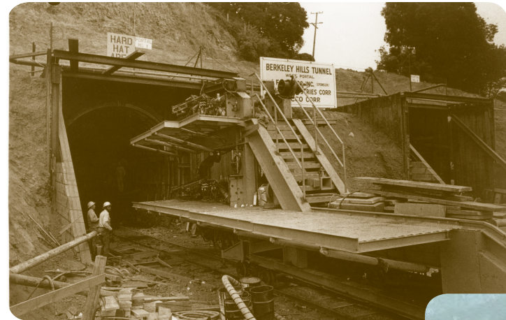
Construction of Berkeley Hills Tunnel.
