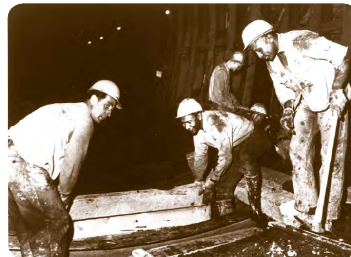
Construction crew in a BART tunnel.
