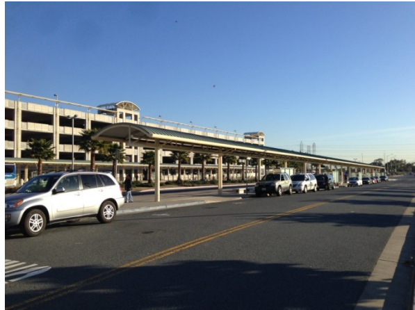
Eastside Pick-Up/Drop-Off Area
