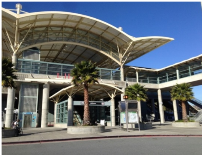
Millbrae Station Eastern Entrance
