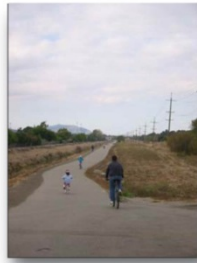
CLASS I BIKEWAY (Bike Path) Provides a completely separated right-of-way for the exclusive use of bicycles and pedestrians with crossflow minimized.
