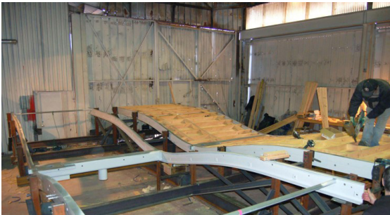
MODULAR CANOPY OFF-SITE PREFABRICATION
