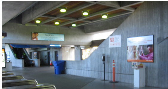
5. South escalator enclosure from west entry
