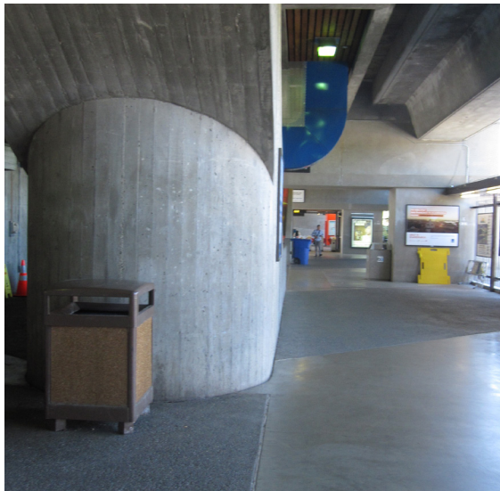
Non-structural concrete escalator surround and bent beyond
