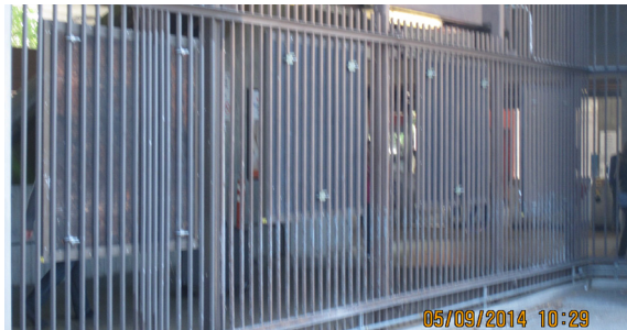
2. West enclosure fence from exterior plaza and bus loop
