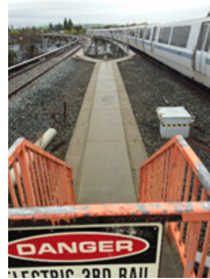
Platform Access Stair at North End of Platform
