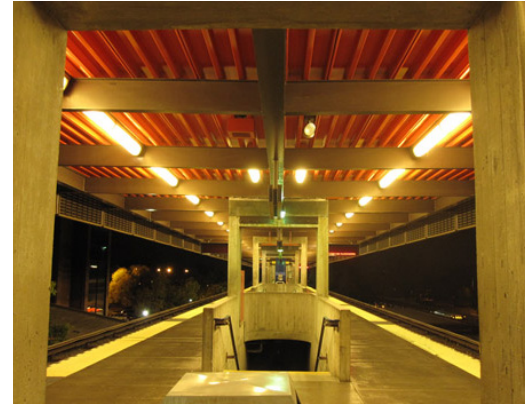
EXISTING CANOPY LIGHTING GLARE
