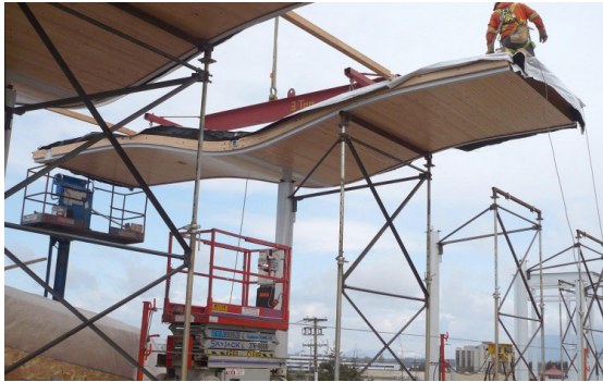
PREFABRICATED MODULAR CANOPY INSTALLATION
