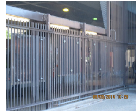
Advertising Panels mounted on Station Enclosure system
