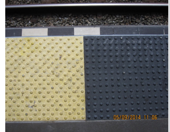
Typical Door Location at Concord is by pattern and color
