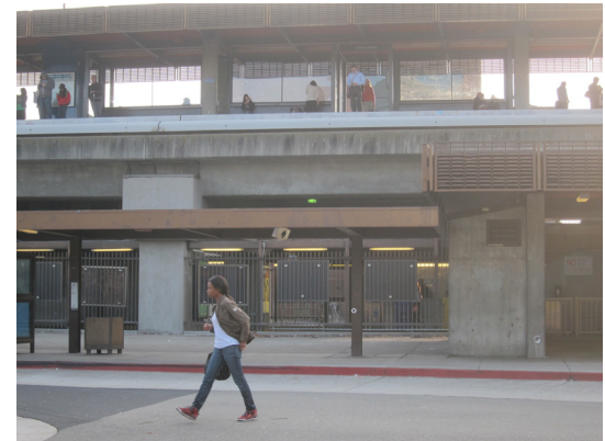
Existing steel grating enclosure with advertising panels
