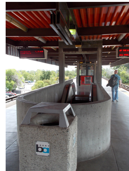
RAW CONCRETE ESCALATOR GUARD
