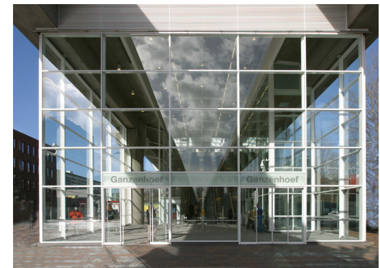
Ganzenhoef Metro Station
