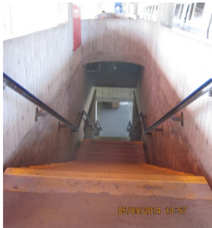
No top of stair tactile warning
