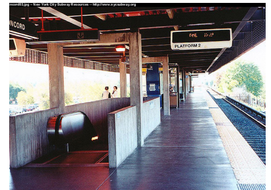
CONCORD STATION 1999-PLATFORM
