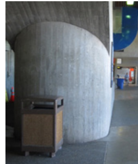
Non-structural, Over-sized Concrete Escalator Cladding
