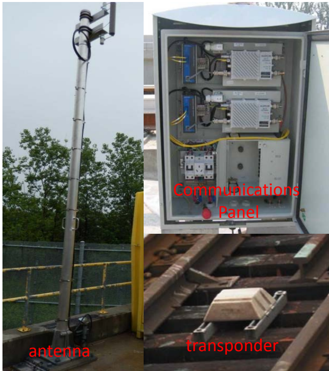
Radio Communications Equipment
