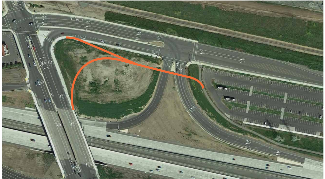
Figure 74 Pedestrian and Bicycle Bridge Across Highway Ramps
