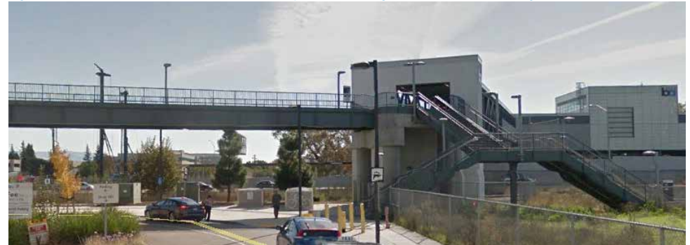
Figure 30 West Dublin/Pleasanton BART station pedestrian bridge and stairs (Source: Google Street View 2016)
