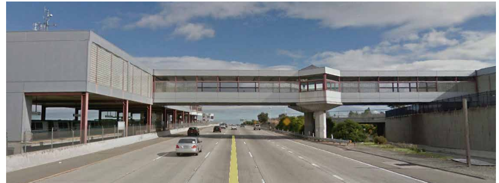
Figure 29 Existing bridge from platform to station entrance and parking lot (Source: Google Street View 2016)
