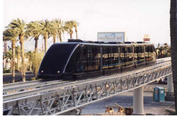
Doppelmyer Cable Propelled System at Mandalay Bay in Las Vegas
