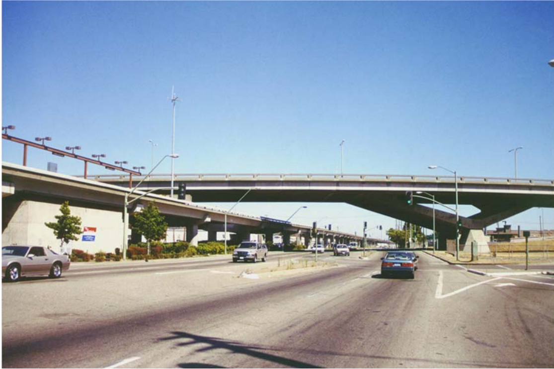
Existing View of Coliseum BART Station (looking east)
