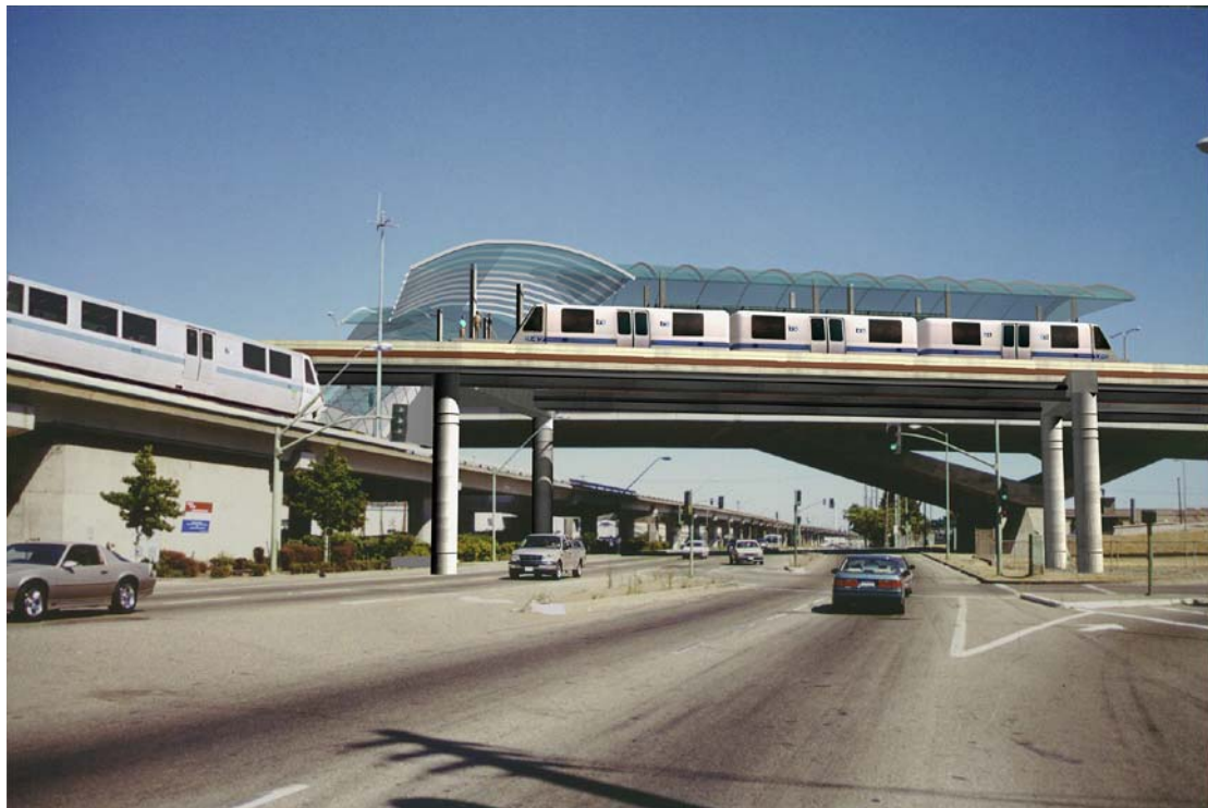
View with Coliseum AGT Station (looking east)
