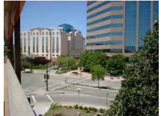
Figure 3.3 – Looking west from the platform at office and hotel development on Oak Street
