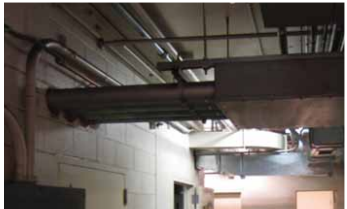
Figure 9: Typical Back-of House lighting)
