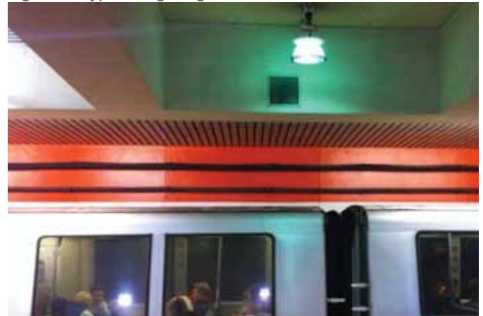
Figure 8: Typical Lighting on the Platform Level
