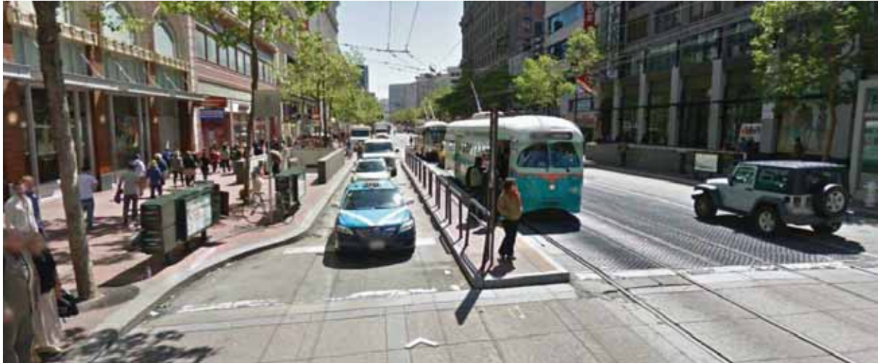
Figure 5 - Typical Air inlet / smoke exhaust grate on Market Street above Powell Street Station
