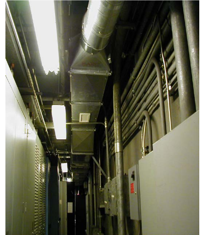
Train Control Room
