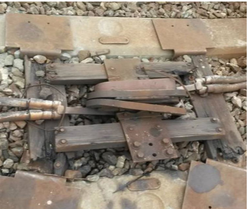
Left: BART's train control system includes both software and hardware, like these "loops," which transmit speed signals to the train. The original core system has 1970's loops, all of which must be replaced. Right: A train control technician at work.
