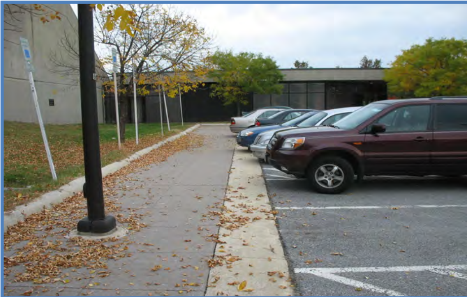
West Hyattsville: Sidewalk location is far from pedestrian desire lines
