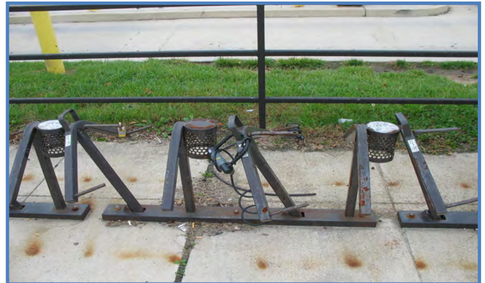
West Hyattsville: Type III bike racks are difficult to use and are often broken
