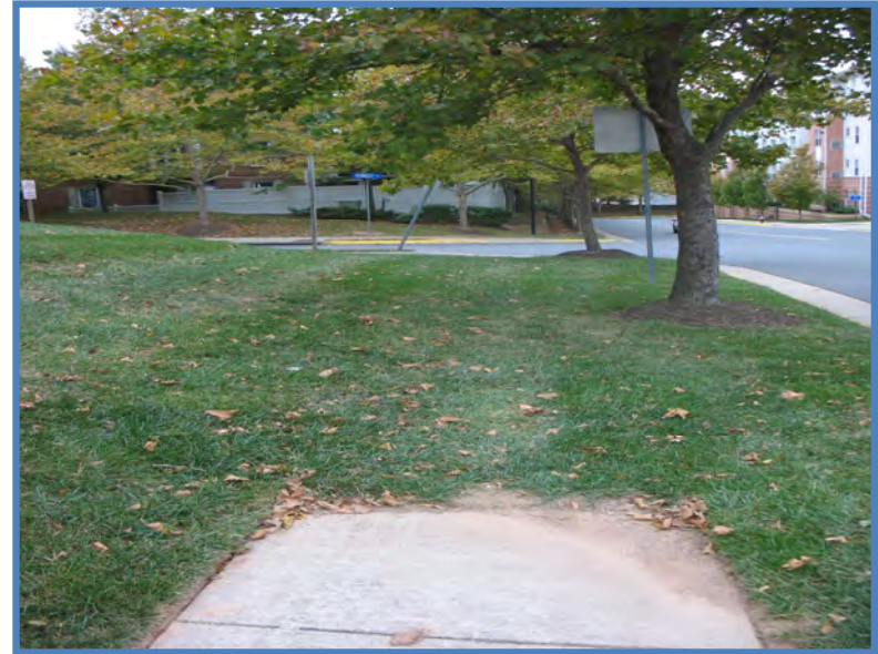
Vienna/Fairfax-GMU: Sidewalk ends at inappropriate place
