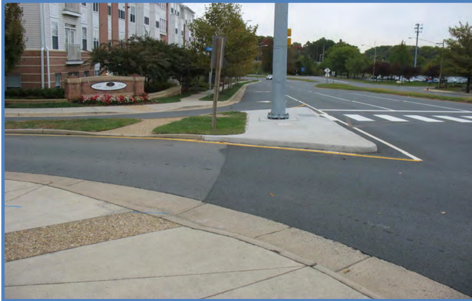
Vienna/Fairfax-GMU: Crosswalk is not ADA compliant
