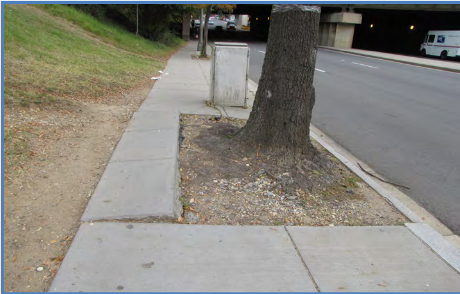
Rhode Island Ave-Brentwood: Sidewalk design is not ADA compliant
