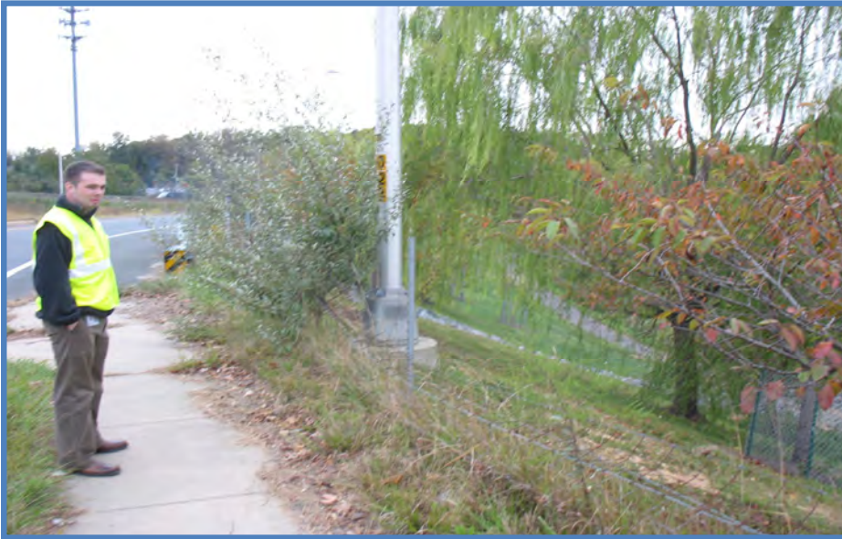
Vienna/Fairfax-GMU: Pedestrian crossing button is obstructed by vegetation
