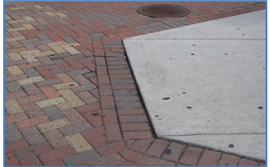
Ballston-MU: Curb ramp is not ADA compliant (lip)
