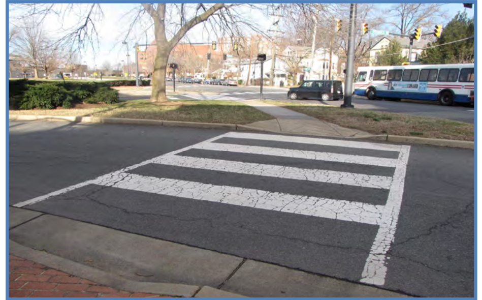
Braddock Road: Curb ramps are not ADA compliant
