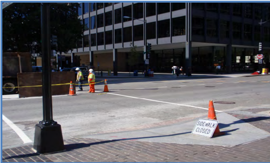
Gallery Place-Chinatown: Construction efforts obstruct pedestrian facilities without detour signage
