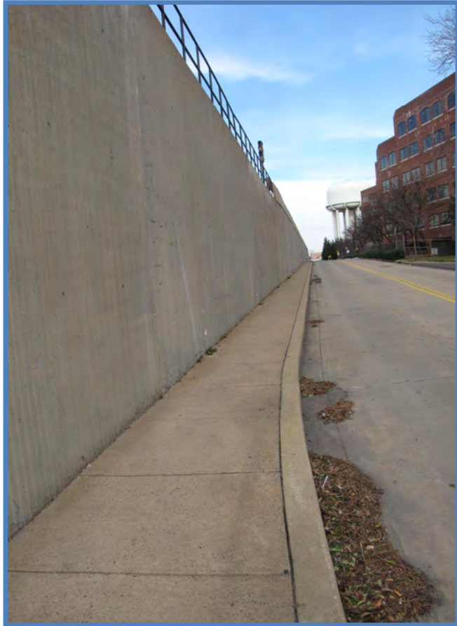
Braddock Road: Narrow and constrained sidewalk
