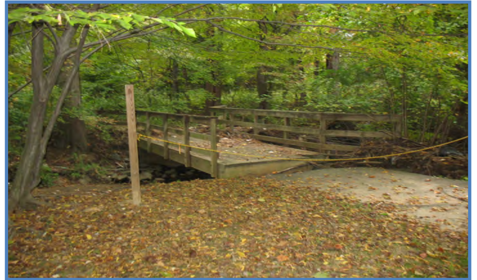
Vienna/Fairfax-GMU: Bike and pedestrian bridge is out of service without further information posted regarding timing or detour
