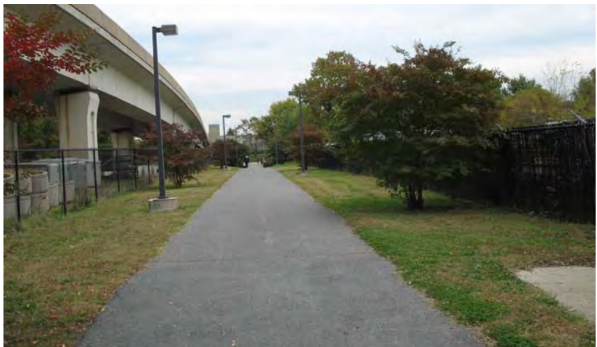
Figure 23: Multi-Use Trail at the West Hyattsville Metrorail Station
