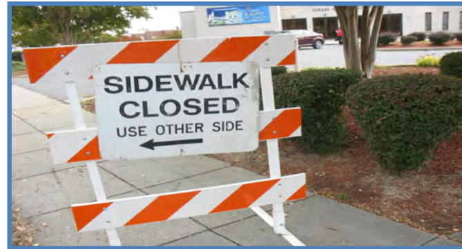
Rhode Island Ave-Brentwood: Construction efforts obstruct pedestrian facilities
