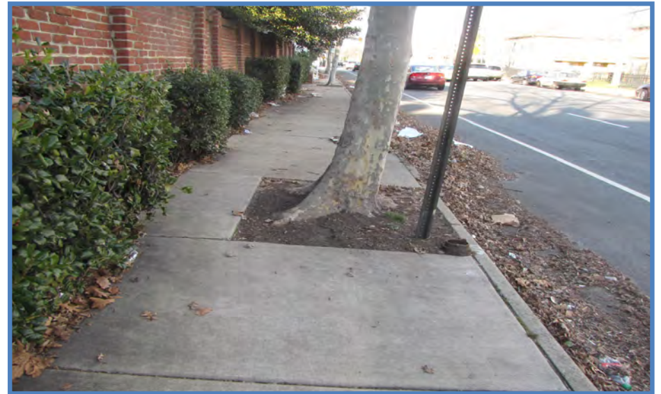
Braddock Road: Sidewalk design is not ADA compliant (physical obstruction)
