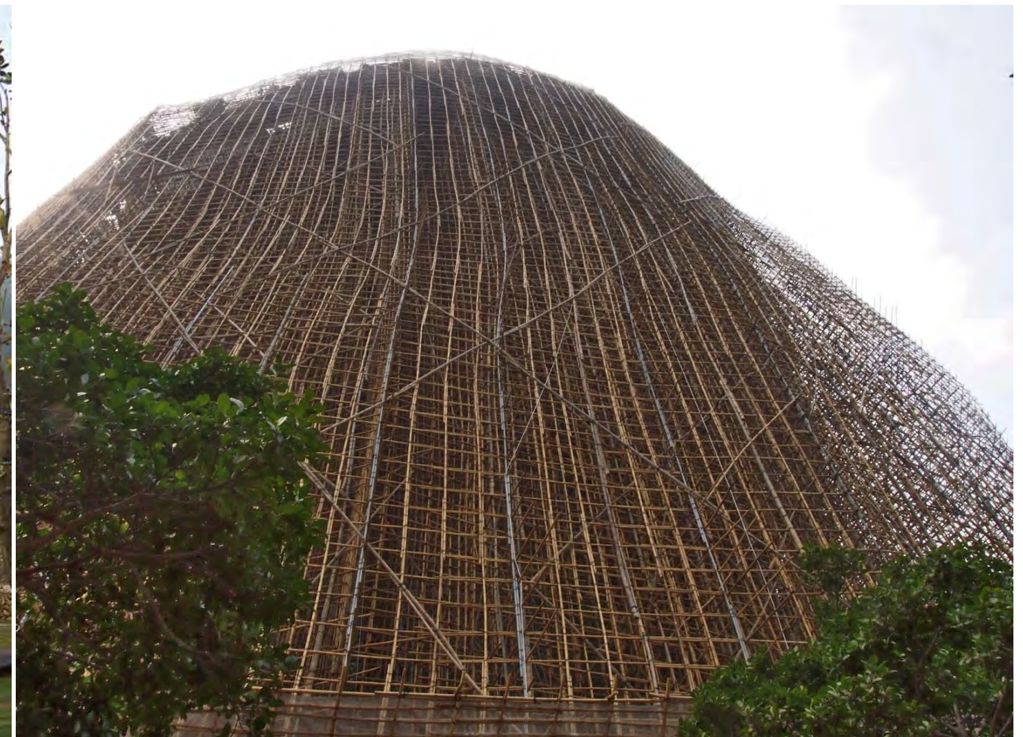
Hong Kong Convention and Exhibition Center, Temporary Scaffolding
