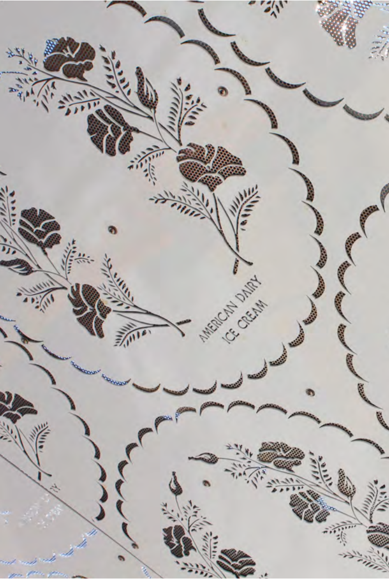
Room Within, San Jose, CA merge conceptual design custom perforated aluminum panels
