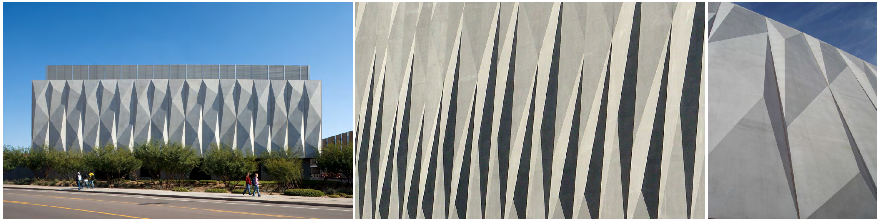
Sun Devil Energy Center at Arizona State University, Tempe, AZ Machado and Silveti Associates
