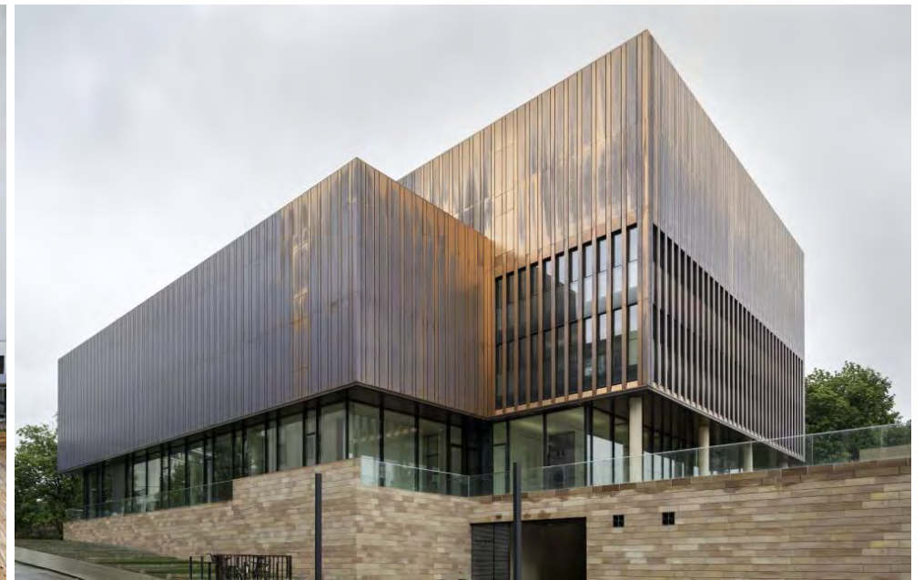
Archive of the Evangelical Lutheran Church of Bavaria, Nuremberg, Germany Gerkan, Marg & Partners Architects Copper Siding, Glass, Sandstone
