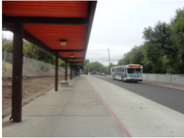
Concord Station's large intermodal center was scaled to meet its role as an end-of-line station. It has been served by fewer bus routes since the BART line was extended in 1996.
