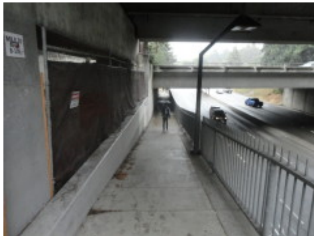
The pedestrian path between the station and theatre is poorly lit and not well signed.
