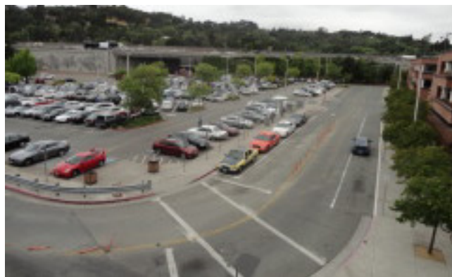
As part of the Walnut Creek Transit Village project, the bus intermodal center will be moved to the west side of the station.
