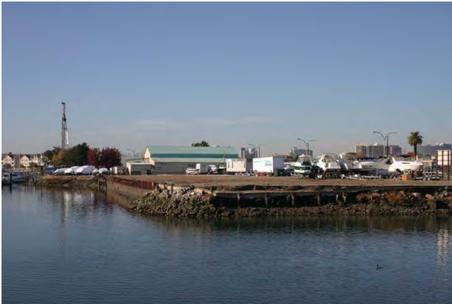
11. Bay Trail Pier looking north
