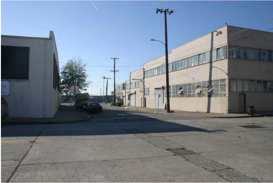
7. East 10th Street at 8th Avenue looking southwest
