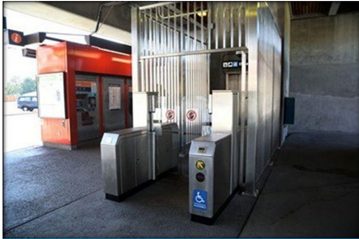
CONCORD (Completed Oct 2020)
