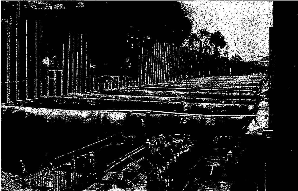
After completing a segment to the north, the contractor began work on the subway south of the South San Francisco station (above). The floor of the subway is being formed and concrete placed in 100-foot-long segments (left).
