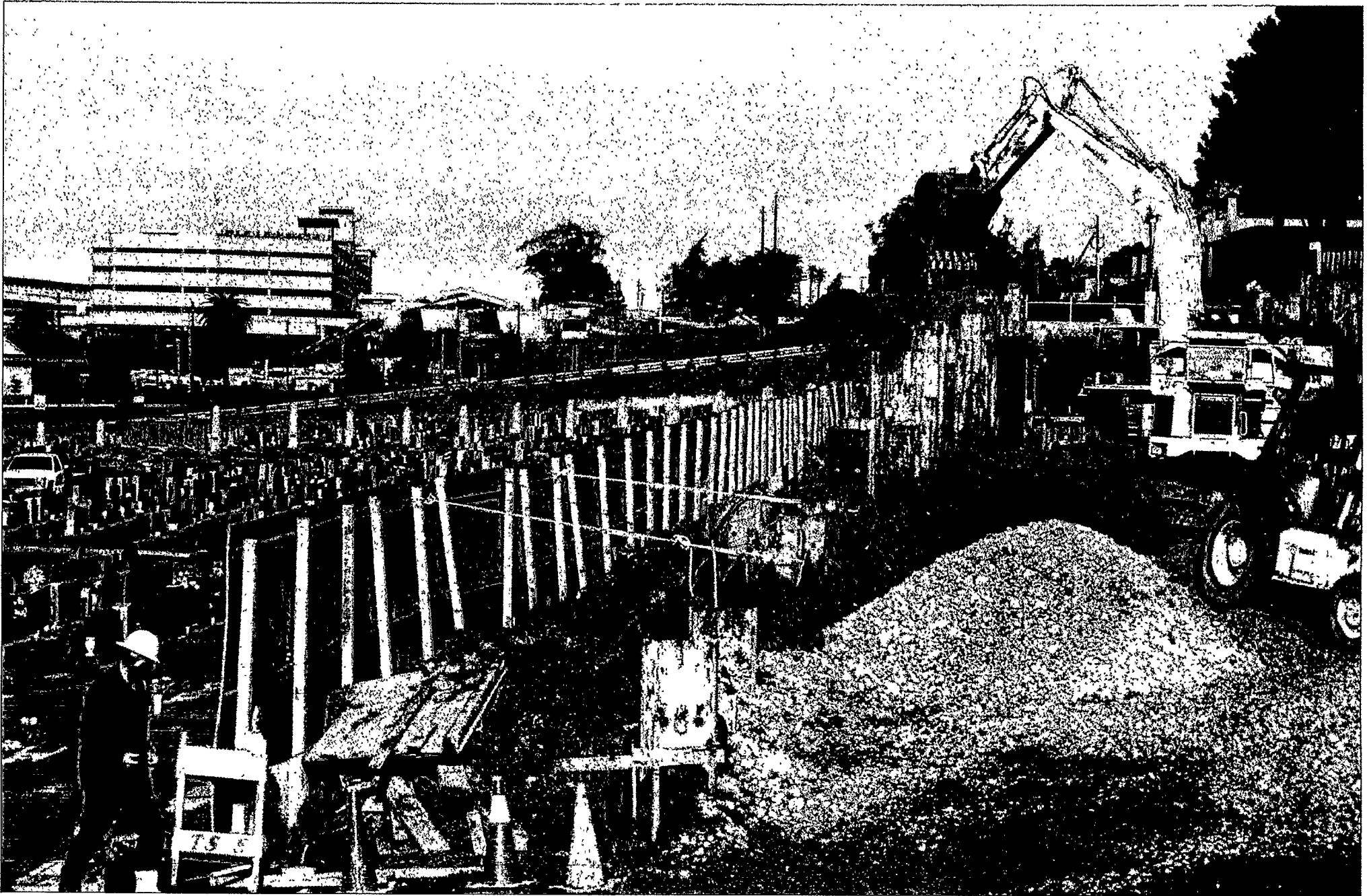
Subway construction through cemeteries with BART Colma Station in background
