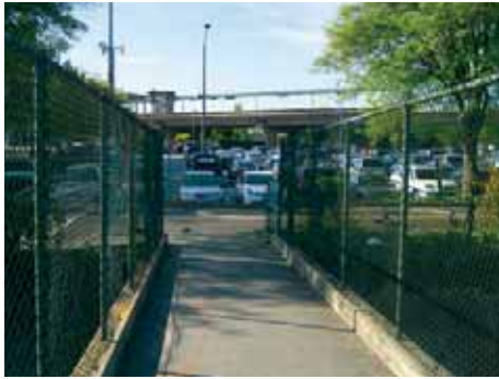
Replacing the existing chain link with the proposed fence will make the bridge experience more pleasant and less confined.
