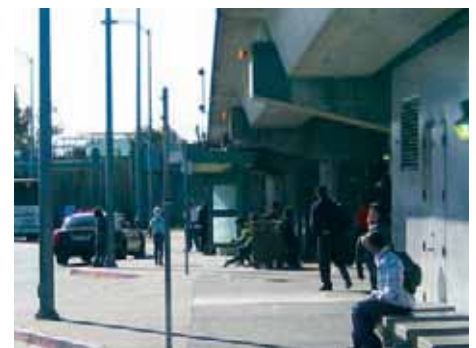
The installation of a new security fence will prevent access to the area underneath the elevated BART tracks.
