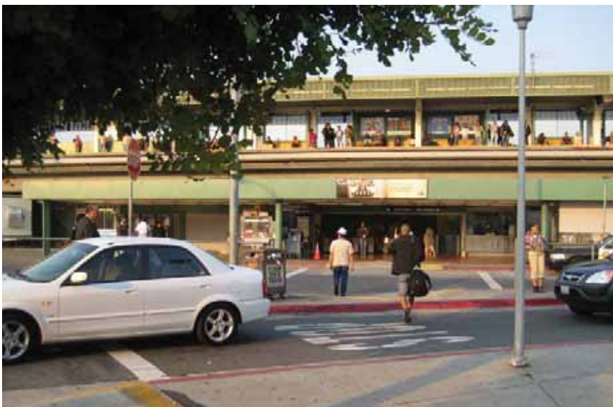
The Bay Fair BART station entrance from the northeast parking lot.
