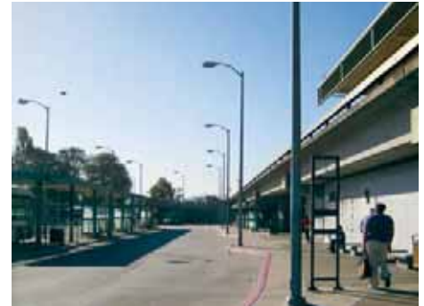
The AC Transit Intermodal Terminal.
