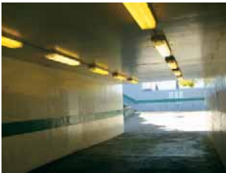
Rehabilitation of the overhead lights in the pedestrian underpass will improve visibility.
