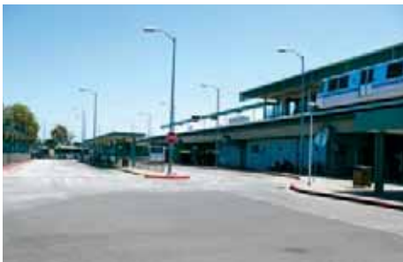
The AC Transit Intermodal Terminal is located adjacent to the station entrance.
