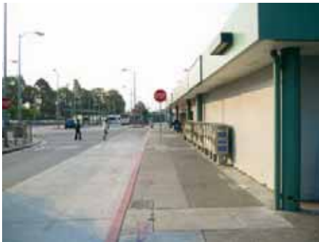
Walls at the station entrance hinder visibility.
