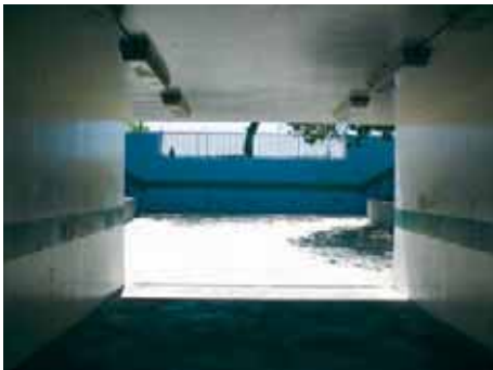
The pedestrian underpass at the Bay Fair BART Station.
