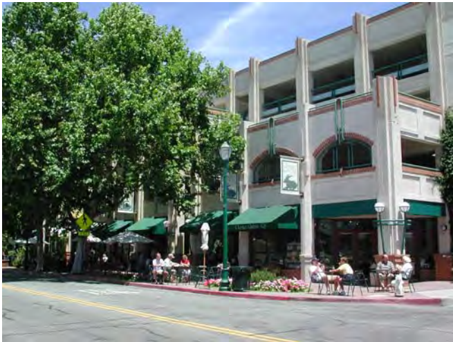
Mixed Use Parking Structure
