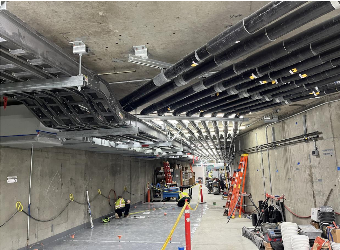
Overhead Raceway and Conduits at Civic Center Substation
