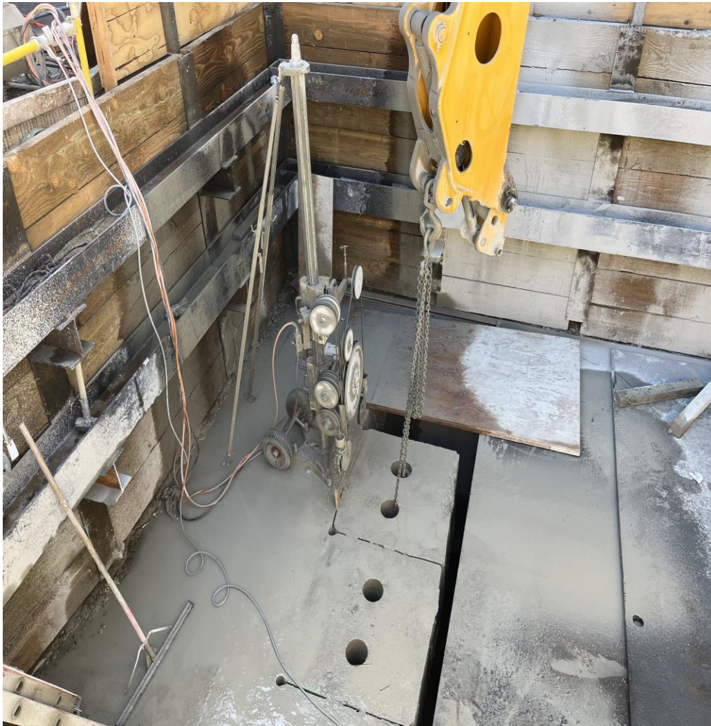
Cutting Concrete to Lower Equipment at Civic Center Substation
