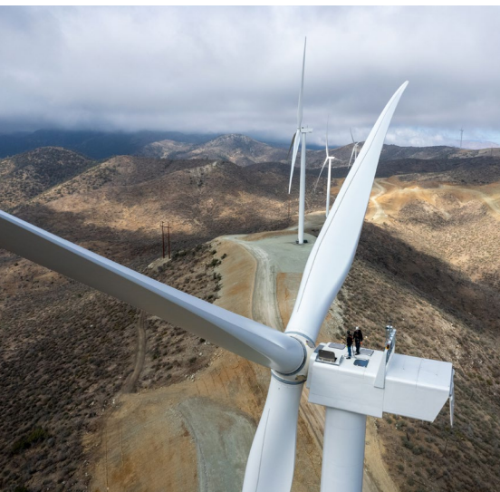
Sky River Wind is a 30-megawatt wind project located in the Tehachapi Mountains. It is a repower project that replaced an older wind project with newer, larger, and more efficient wind turbines. Pictured here are Paul Bostrom, BART's Energy Division Manager, and a NextEra Energy Resources technician standing atop a turbine. Photo courtesy of NextEra Energy Resources.
