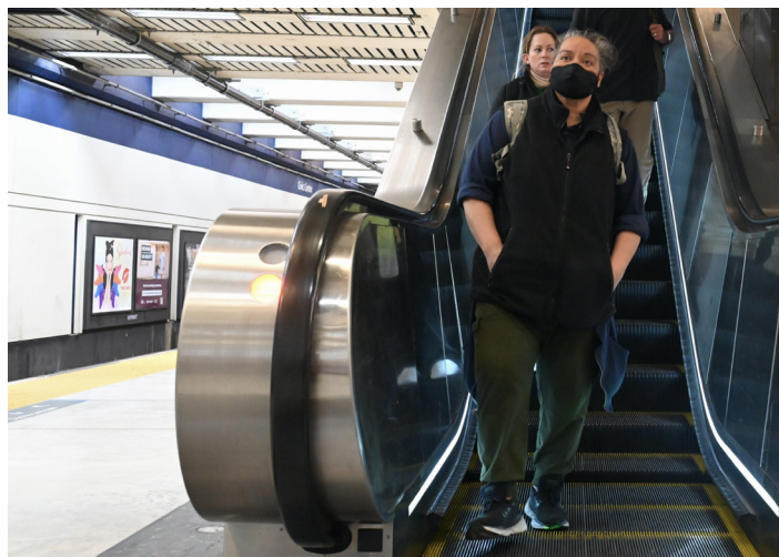
BART's new escalators are more energy efficient, with LED lighting, a "sleep mode," and variable frequency regenerative drives.
