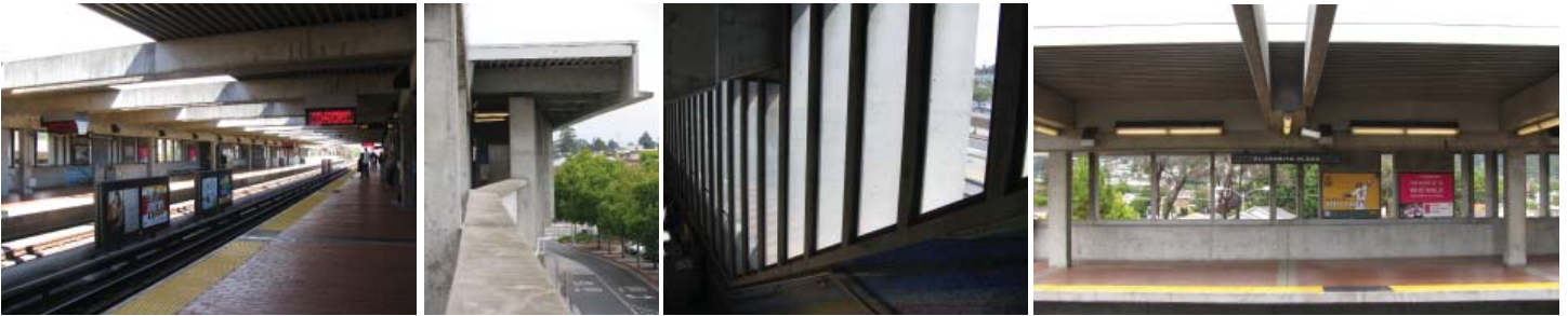
Repetitive, concrete structure creates hierarchy of form, space and order.
