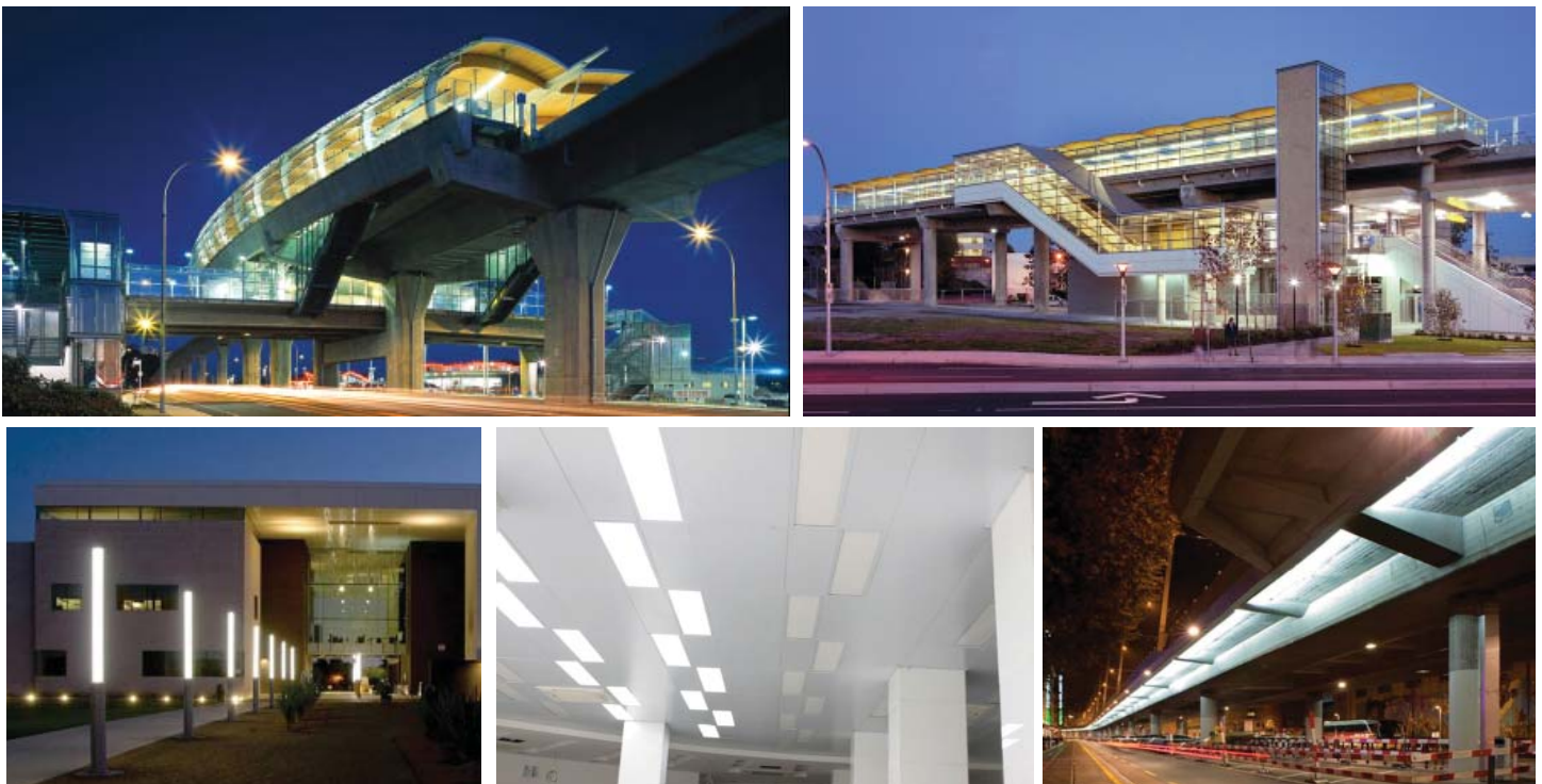
Site lighting, station lighting and metal ceiling LED lighting systems.
