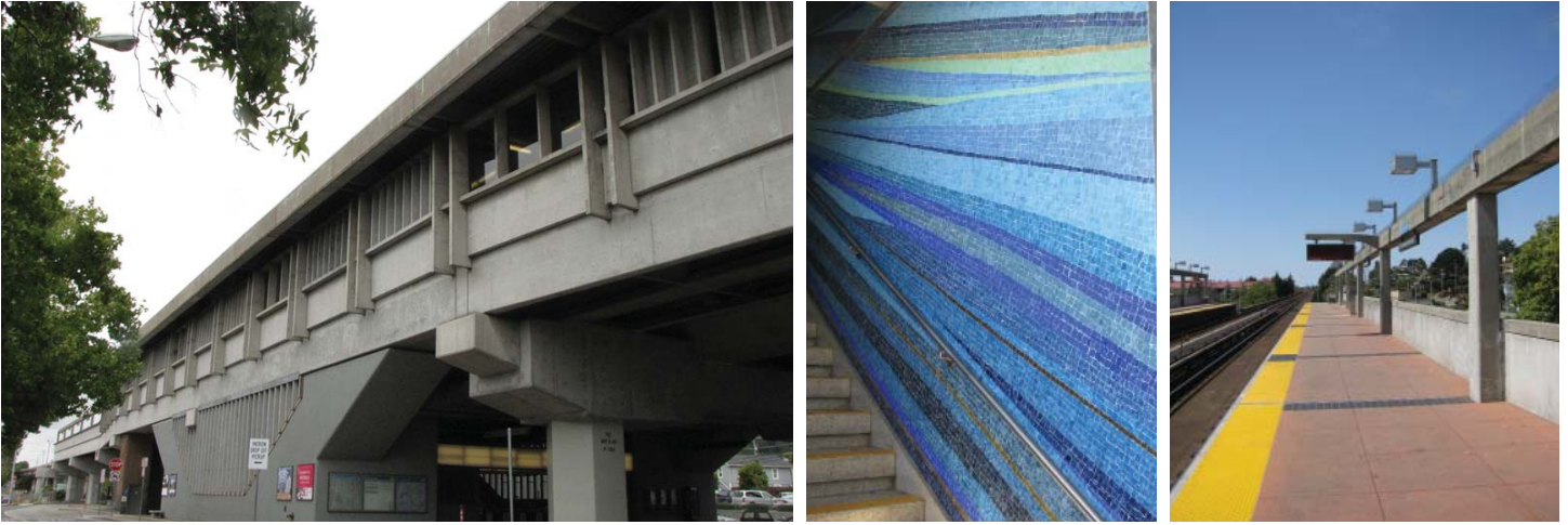
Rhythmic motif of vertical fins, mosaic tile artwork, structure framing view of surrounding hills.
