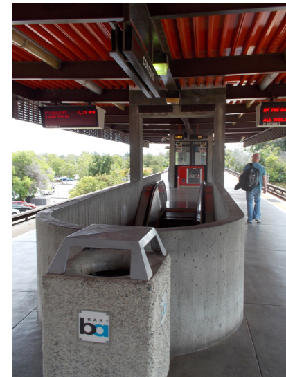
RAW CONCRETE ESCALATOR GUARD
