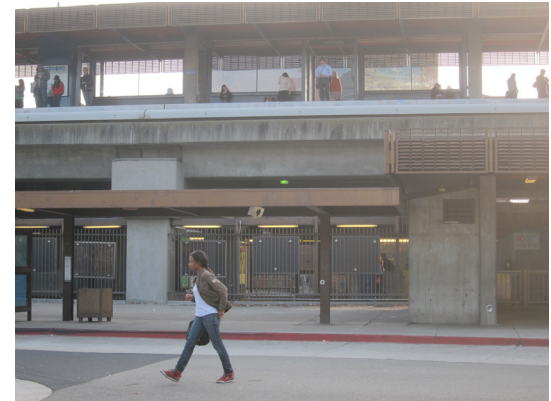
Existing steel grating enclosure with advertising panels
