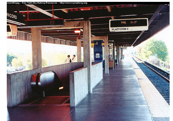
CONCORD STATION 1999-PLATFORM
