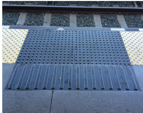
The four enter platform door locations include directional tactile information panels
