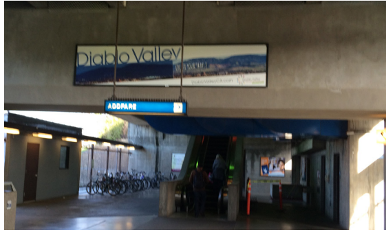
4. SP 42 facing north escalator
