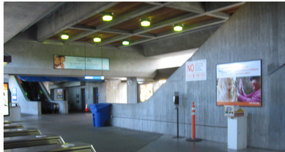
5. South escalator enclosure from west entry
