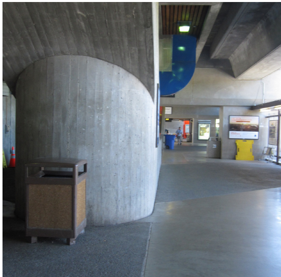
Non-structural concrete escalator surround and bent beyond
