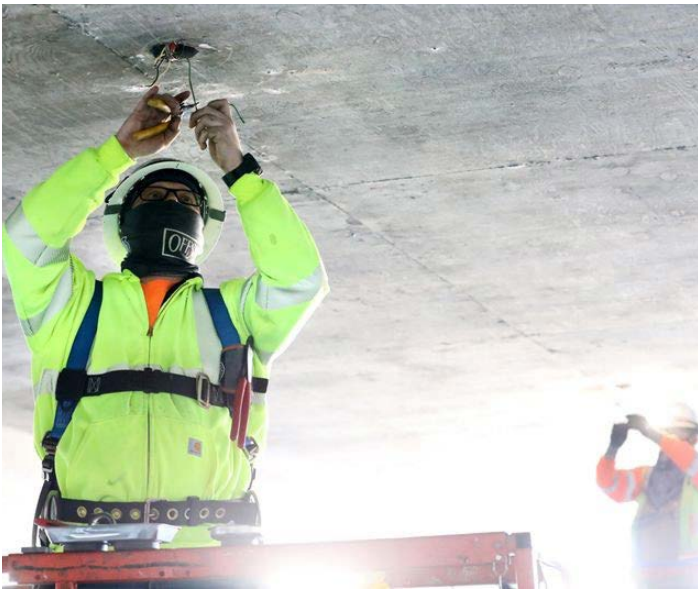
BART replaced the lighting at 14 of our 15 parking garages several years ago. The new LED lights are more energy efficient, last longer, and are brighter than the previous lights.
