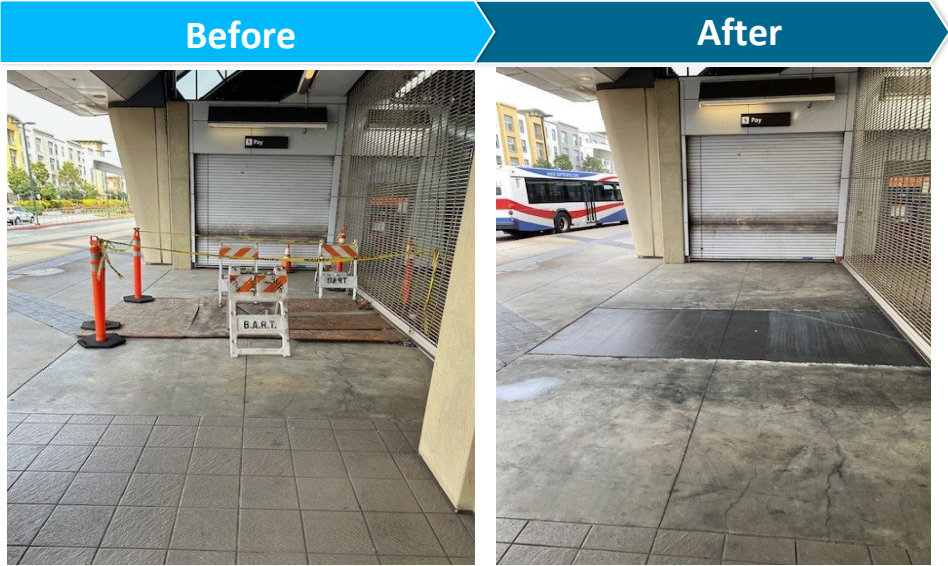
South San Francisco: Repaved Uneven Concrete Pavement
