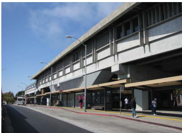
Southwest view of El Cerrito del Norte Station
