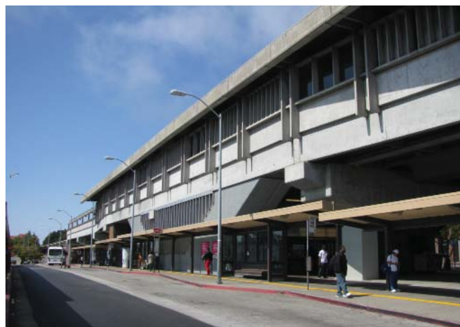
Southwest view of El Cerrito del Norte Station
