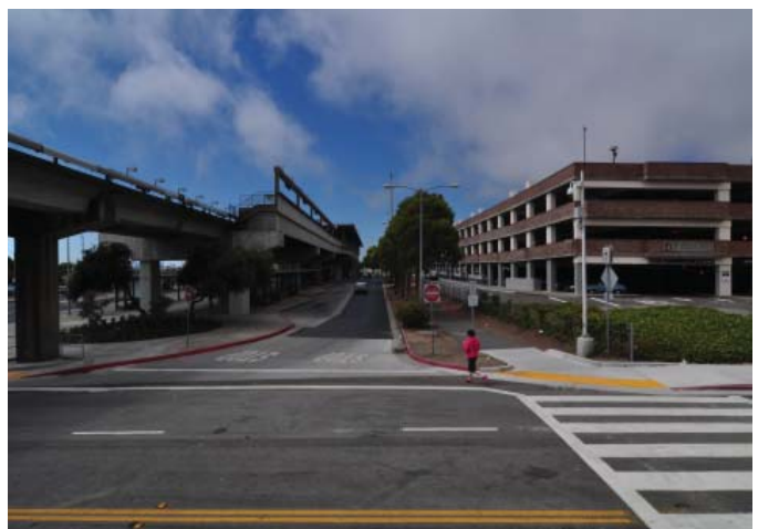
Del Norte parking structure, Ohlone Greenway and intermodal road
