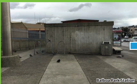
Existing station conditions
