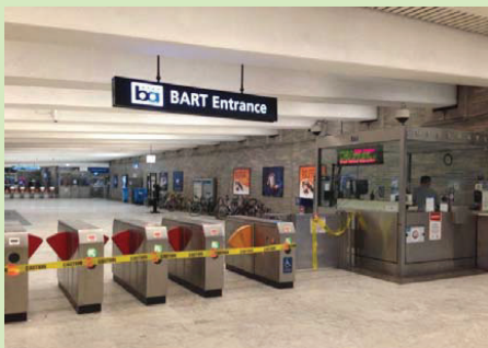
Aging station components and infrastructure lead to periodic service disruptions.
