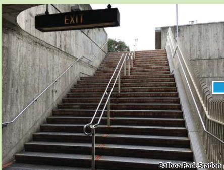
Existing station conditions
