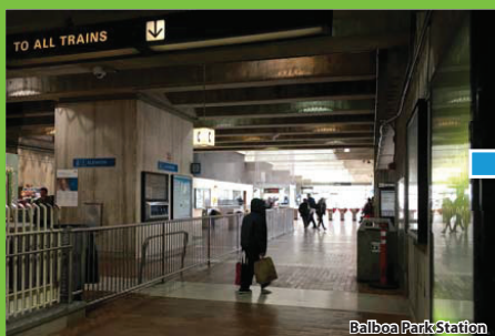
Existing station conditions
