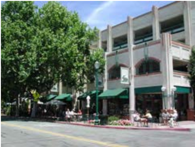
Mixed Use Parking Structure
