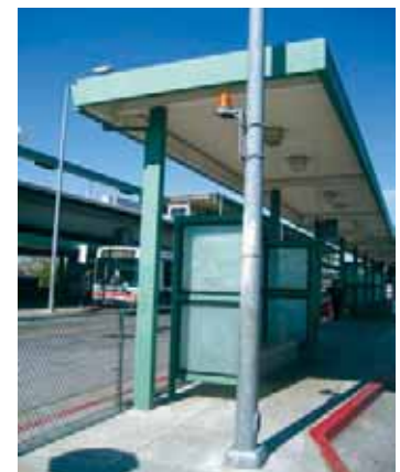
The non-transparent wind shelters hinder visibility in the AC Transit Intermodal Terminal.
