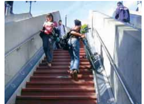
Bicycle stair ramps will improve bicycle access through the pedestrian underpass.
