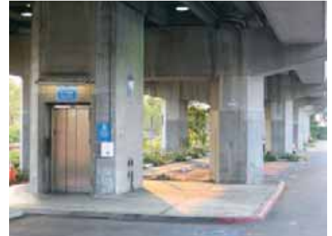
The elevator is isolated and hardly visible from the station fare gates.
