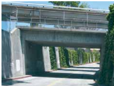
Bikes and Pedestrians are prohibited on the Thornally Drive underpass.
