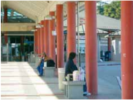
The bus bays at the North Concord BART station transit stop are open and provide visibility.
