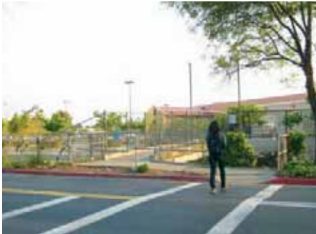
The pedestrian bridge over the Estudillo Canal.
