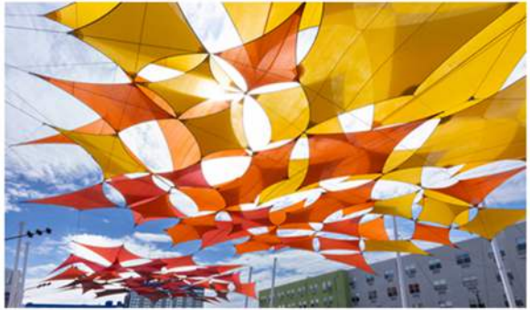
OVERHEAD SHADE STRUCTURE
