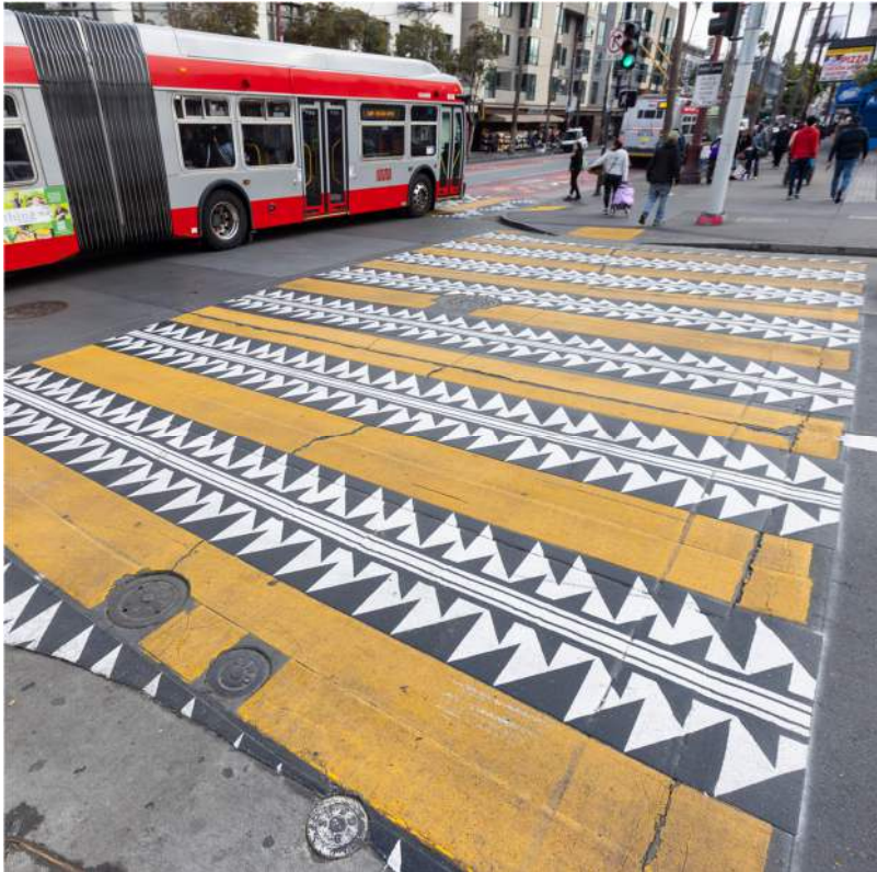
AICD-LED CROSSWALK TREATMENT
