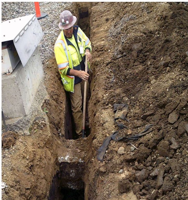
Construction Crew at the Hayward Yard
