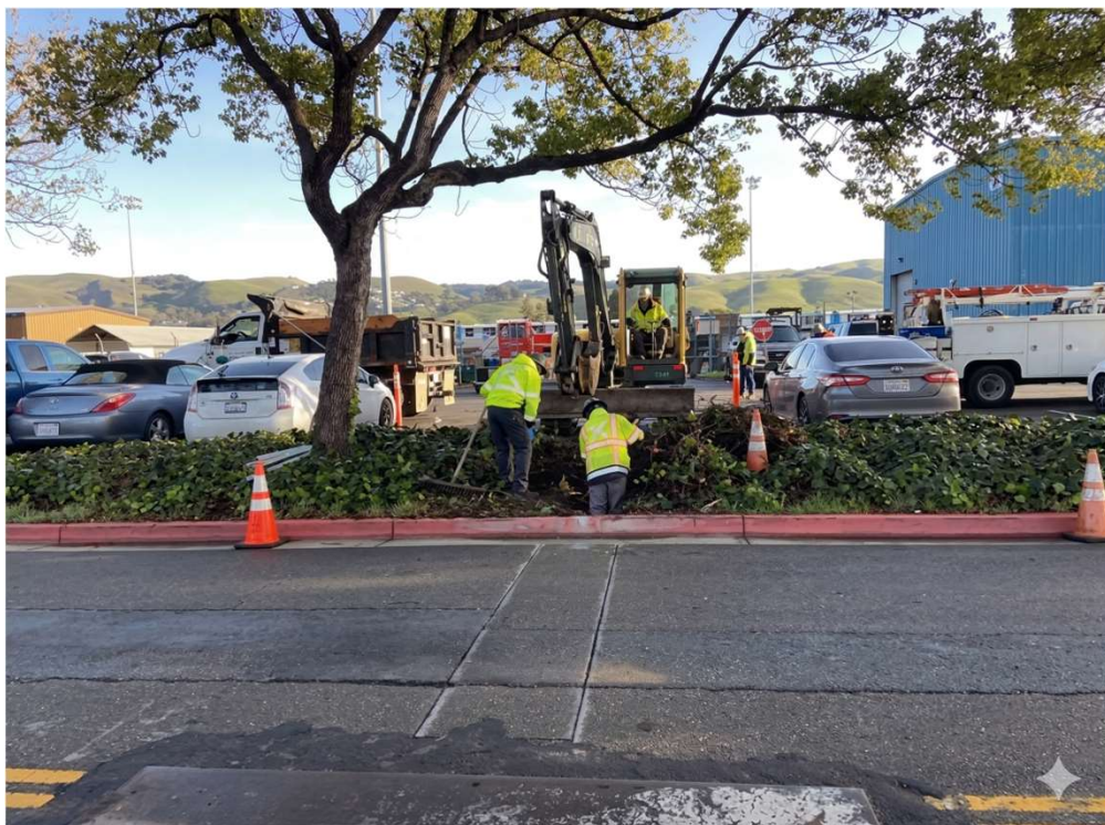
Construction Crew at the Hayward Yard
