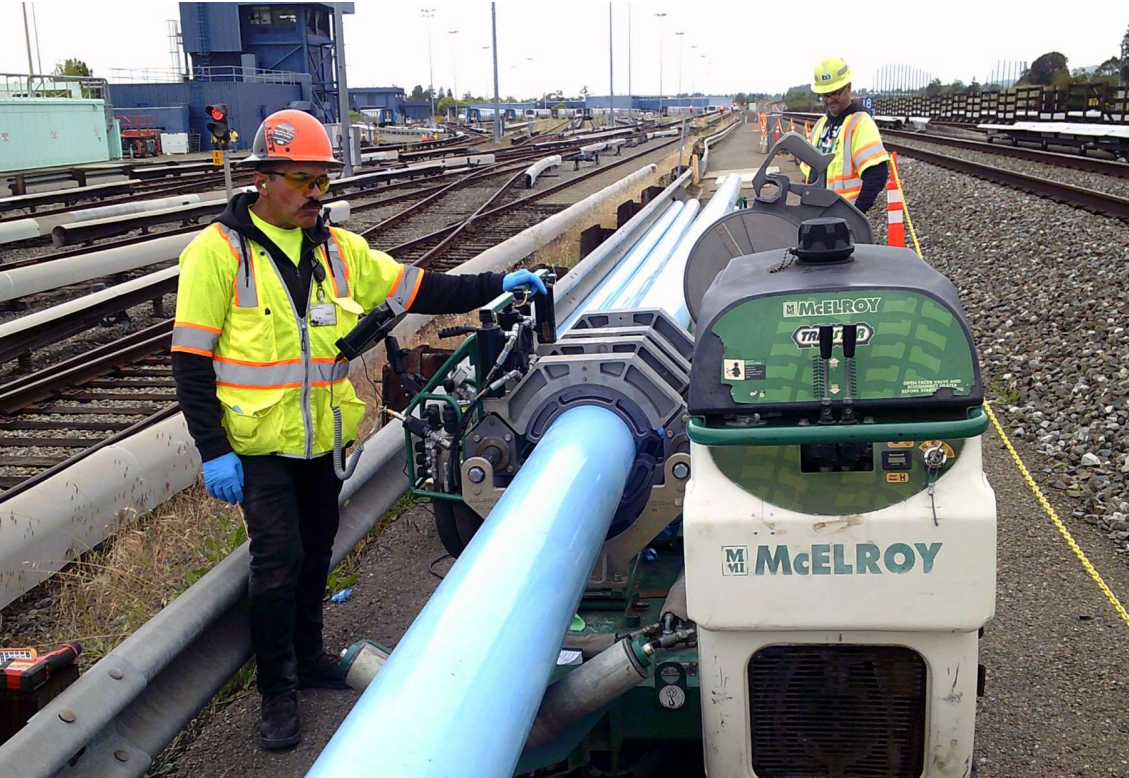
Construction Crew at the Hayward Yard
