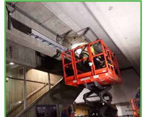
Began installation of 6"x4" cable tray on the girder adjacent to M2 track
