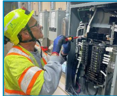
Power Panel installation at Colma
