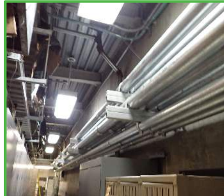
Continued installation of new conduit in the Daily City Train Control Room
