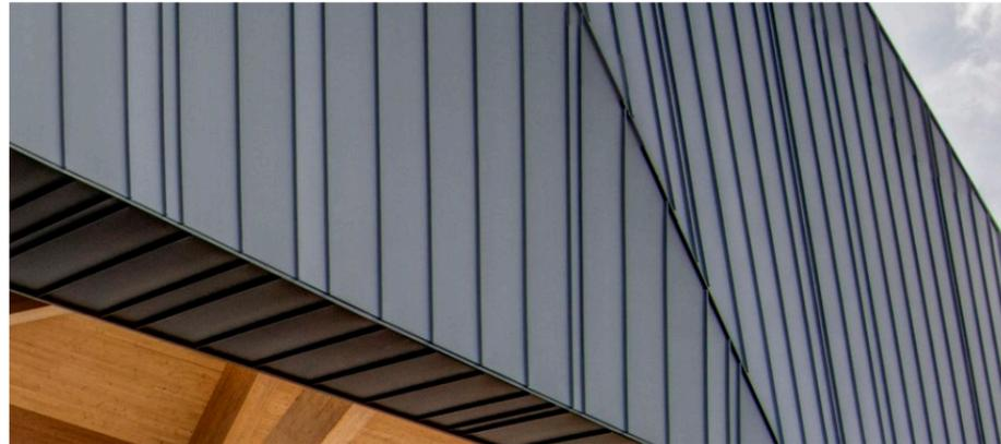
**Zinc alloy standing seam metal cladding:** standing seam metal is an extremely durable roof materials that can also be used for wall cladding. It is expressive of traditional craft yet can be used to clad contemporary, sculptural forms. The dark, neutral coloring of zinc alloy is both contemporary and neutral, and complements both the concrete of the existing station structure and the stucco and brick of the Transit Village.
