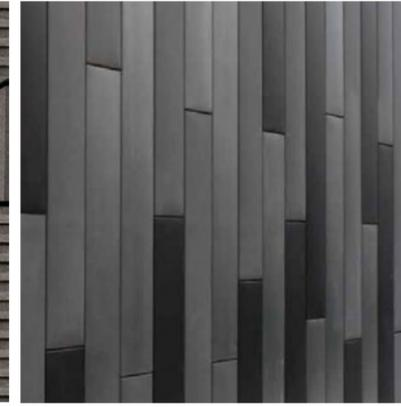
**Other cladding considered:** To the right are alternative cladding materials considered (from left): textured glass fiber reinforced concrete (GFRC) panels, precast concrete panels, and composite metal panels. Each of these can be attractive alternatives to the standing seam metal panels, but are likely to require a more robust structural wall system to support it.
