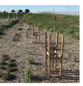
The bioretention areas help capture stormwater and trap pollutants in the soil and roots of vegetation, where they can be broken down by bacteria.
