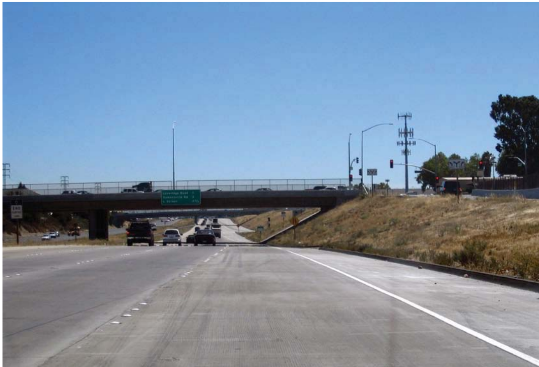
B Eastbound view approaching Railroad Avenue overpass
