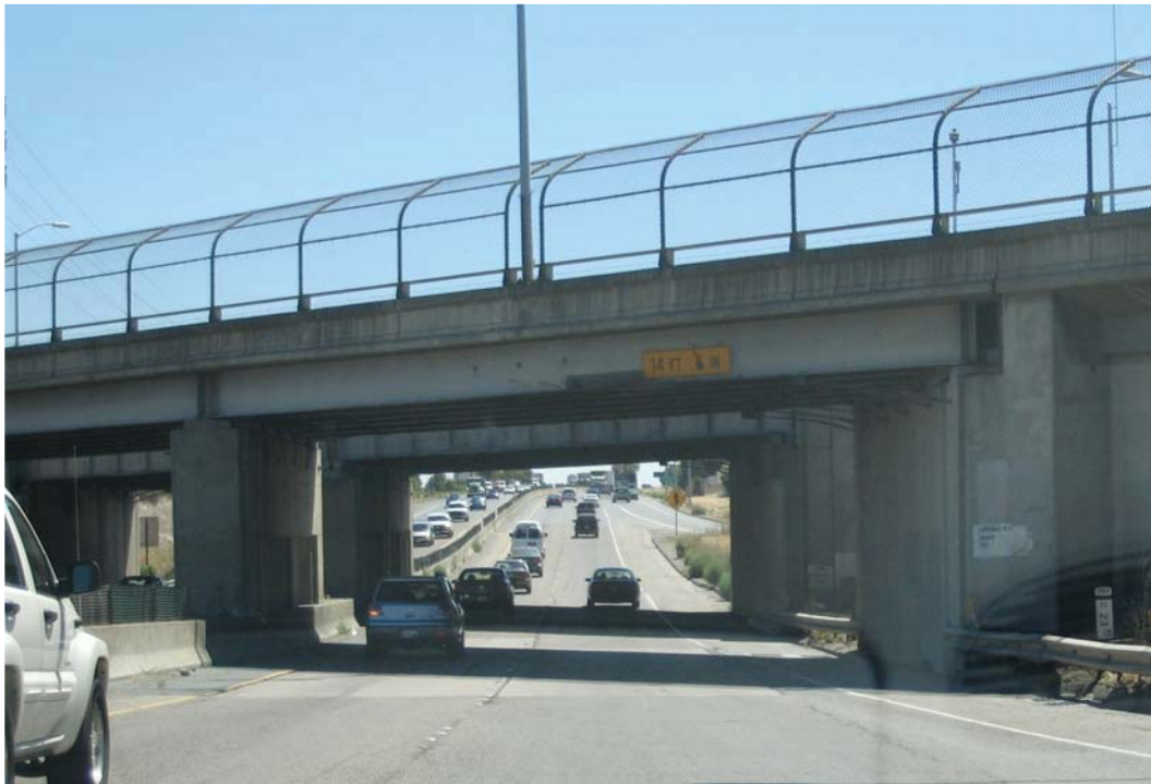
B Eastbound view approaching Loveridge Road overpass
