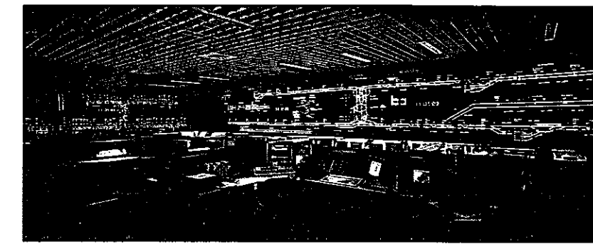
BART Central—the nerve center of the system.
