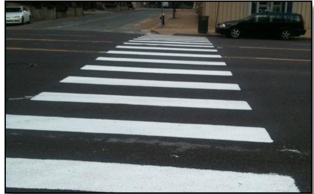
Continental high-visibility crosswalk striping
