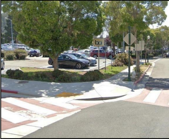
Directional curb ramps
