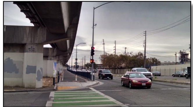
Location of Recommendation PB1: BART columns alongside East Bay Greenway
