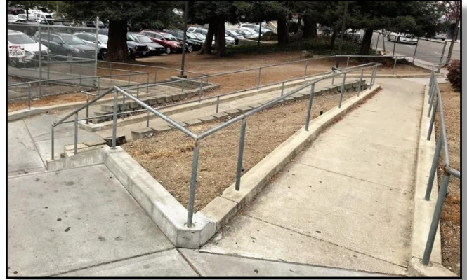
Location of Recommendation P1: Ashby Avenue/ Adeline Street
