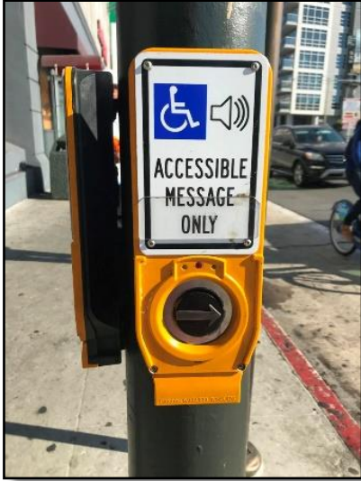
Accessible pedestrian signal
