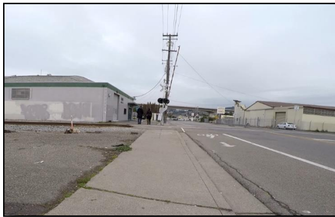
Location of Recommendations P 4 and P 16 : Williams St at UPRR
