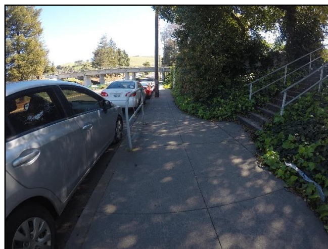
Location of Recommendation P6: Tennyson Road narrow sidewalk
