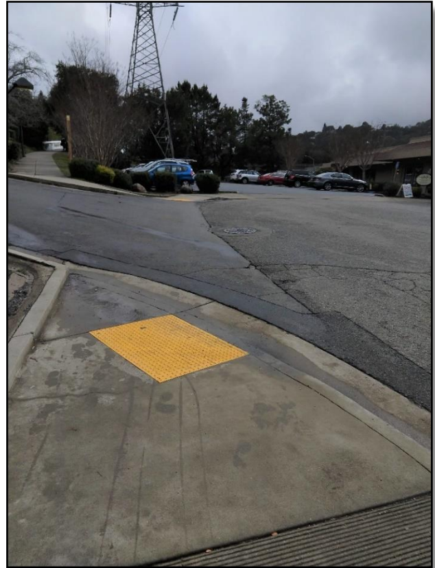
Location of Recommendation P6: South end of Orinda Way
