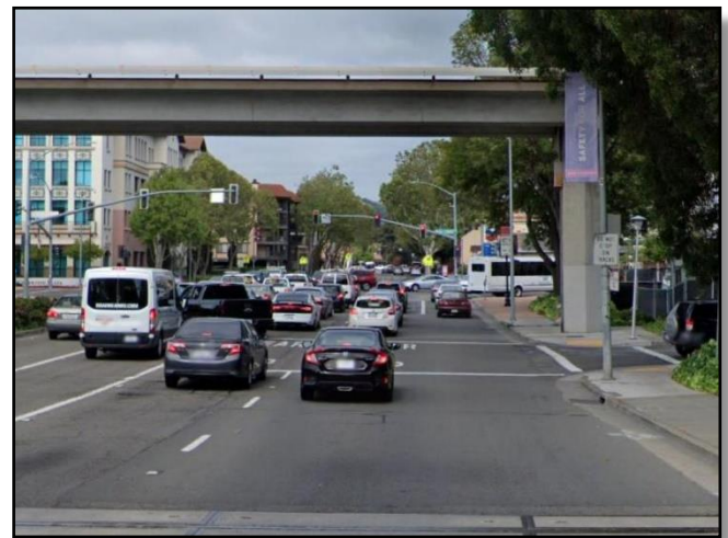
Location of Recommendations P10 and B2: Davis St between Alvarado St and San Leandro Blvd
