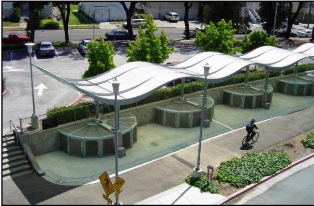
Existing bicycle lockers along Ohlone Greenway
