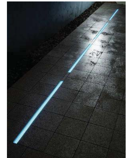
BART blue In ground led strip lighting
