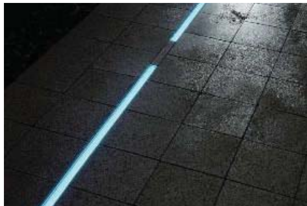
BART blue in-ground lights
