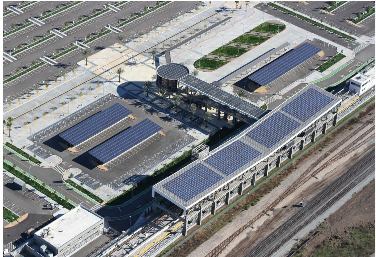
throughout the day, and have the capacity to produce over 500 kilowatt-hours, more than enough to meet the station's daytime power needs. Excess power will be fed back into the gird and will "run the meter backwards." Solar design, installation, and connec-
