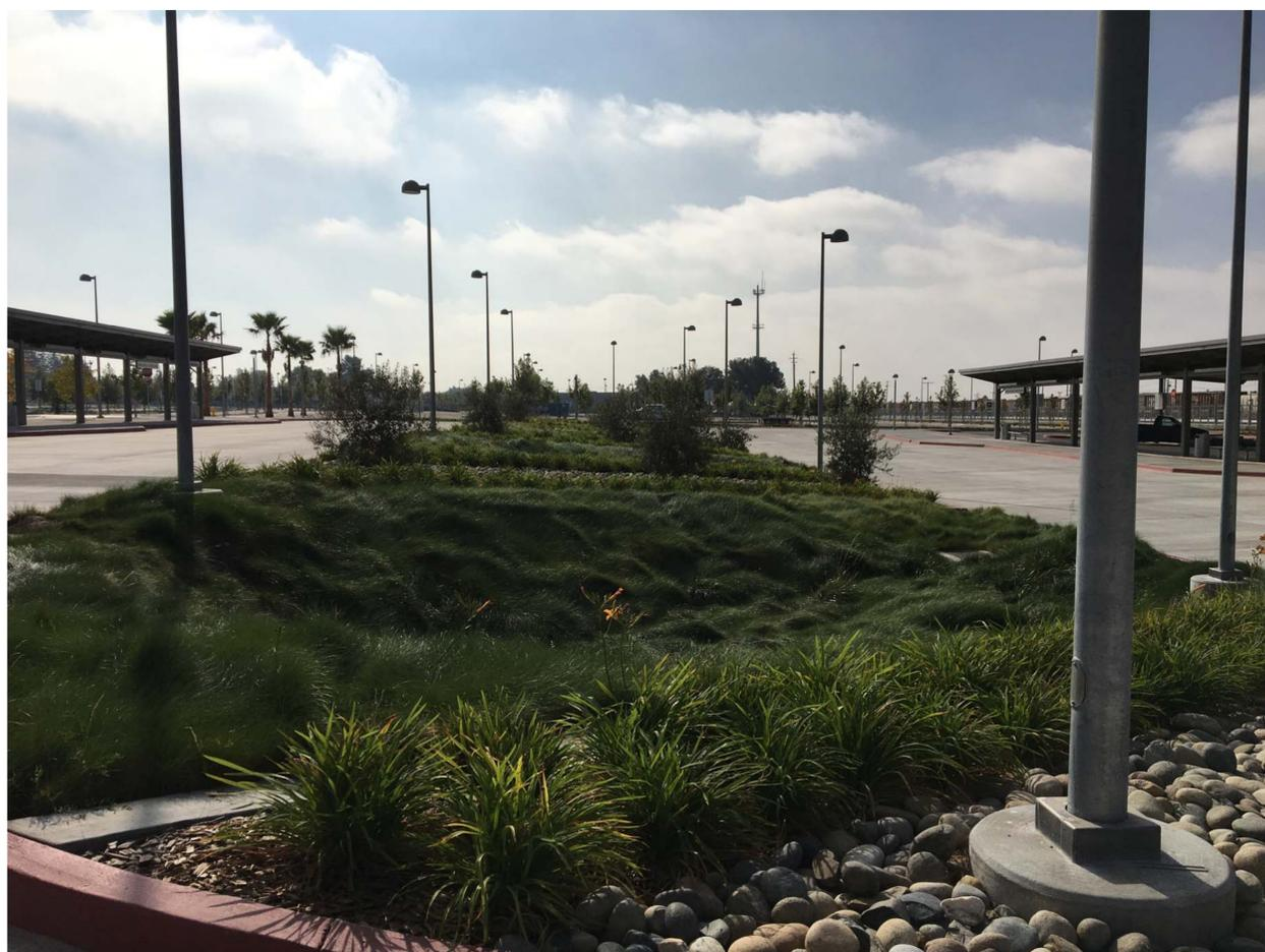
*U-shaped bioswales at Warm Springs/South Fremont Station serve to filter storm water.*
