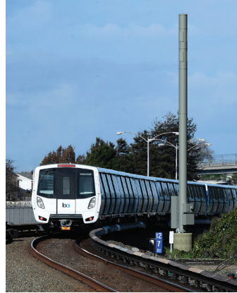
Joint use pole
